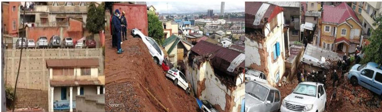
Figure 8: Photo of the parking lot and the house in the capital before and after the landslide (Source: BNGRC, 2022)
