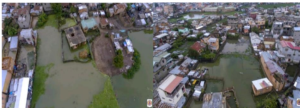
Figure 7: Photo of rising waters after Cyclone ANA in January 2022 (Source: BNGRC, 2022)
